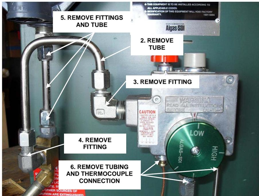
*Figure 2. Disconnecting tubing and connections from Robert Shaw thermostat assembly*
